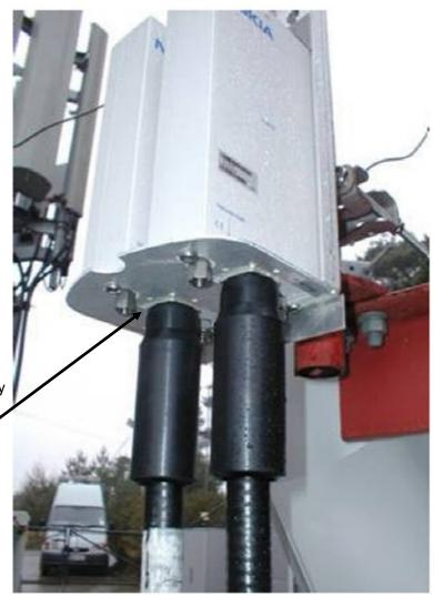
Install: Note correct connector and socket body fully covered with no top gap between device and GCA2.
